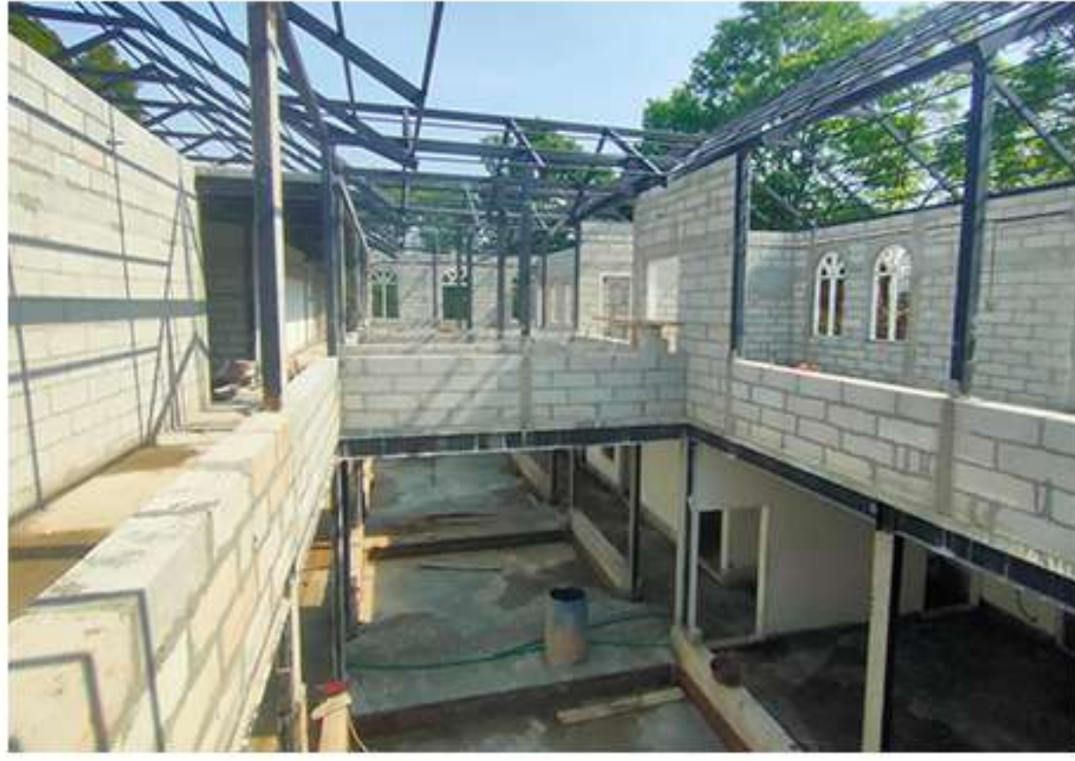
STEEL STRUCTURED CONVENT BUILDING AT THRISSUR
