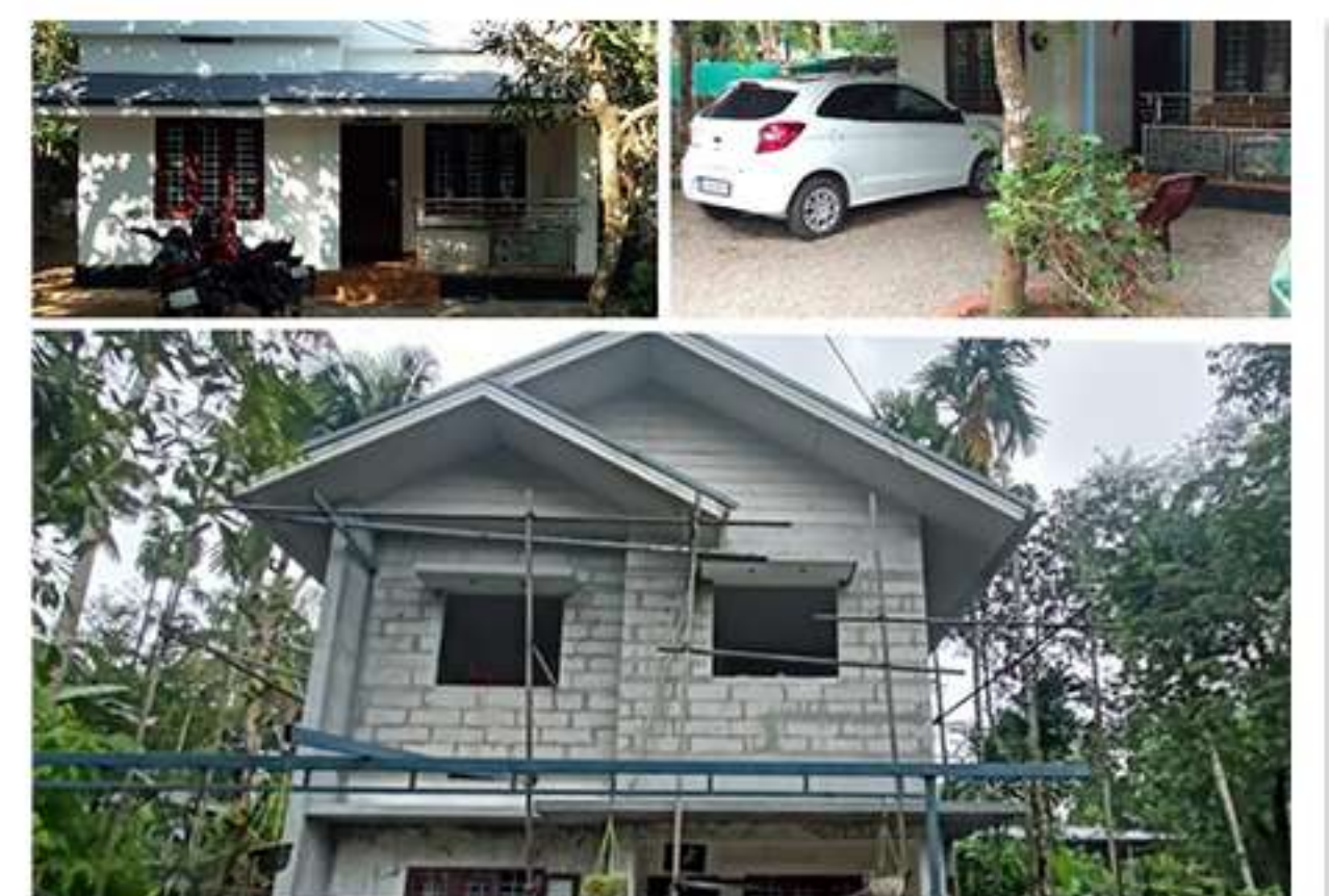
RENOVATION AT THRISSUR
