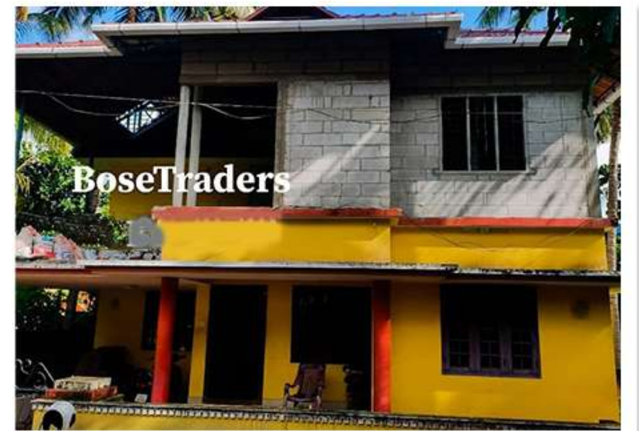
RENOVATION AT THRISSUR
