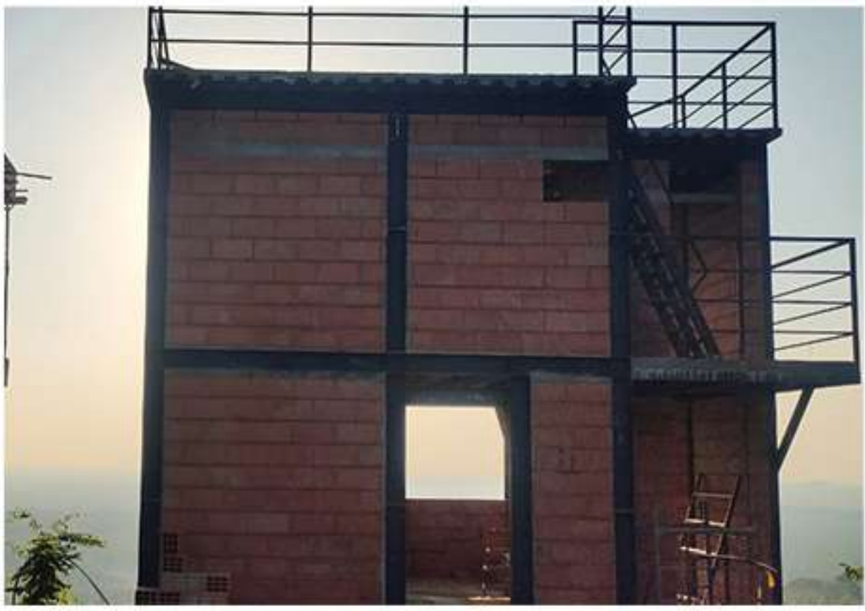
STEEL STRUCTURED RESORT BUILDING
